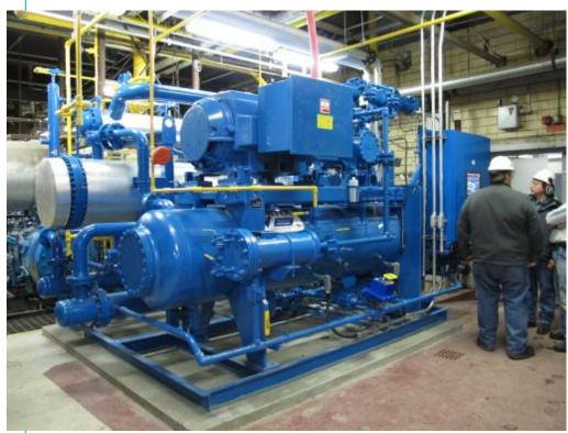
VSSH-451 at 66°F to 86°F Suction Delivering 170 GPM Water at 145°F Saving +\$31/hour
