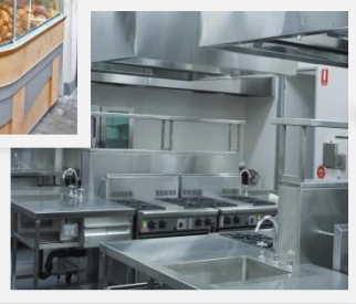
Hot water for sanitary purposes
