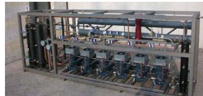
Prodega Givisiez, Switzerland, medium temperature installation, Q'_0 = 150 \text{ kW}
