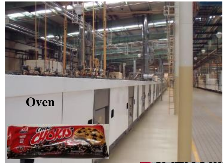
Waste heat recovery Heat exchanger
