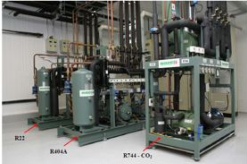
Figure 01: Detail of the refrigeration racks from the CO 2 Technology & Training Center of Bitzer Brazil.
