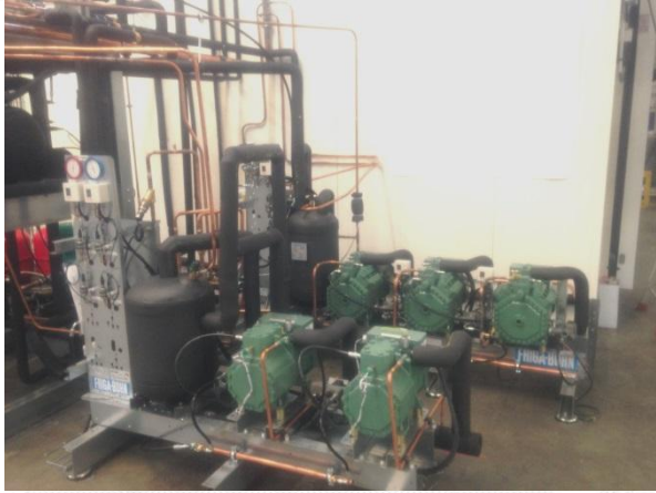
Transcritical Booster System with Parallel Compression for Supermarkets
