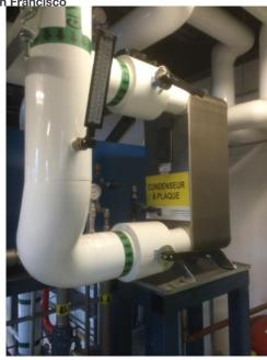
AlfaNova plate condenser U-turn evaporator 71 TR Charge :168 lbs, or 2,4 lbs/TR
