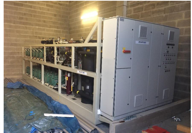
Compressors and Liquid receivers side
