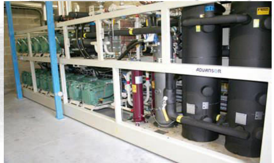
Compressors and Liquid receivers side
