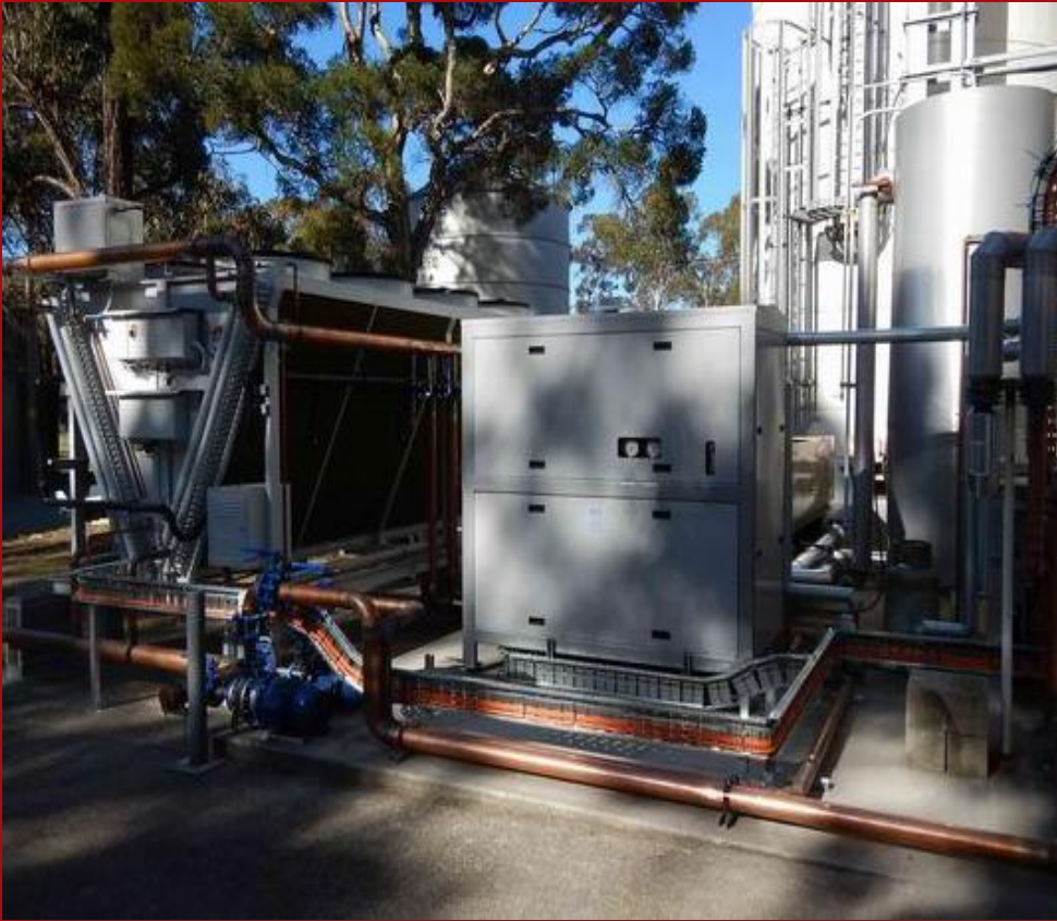
Chiller and remote dry cooler
