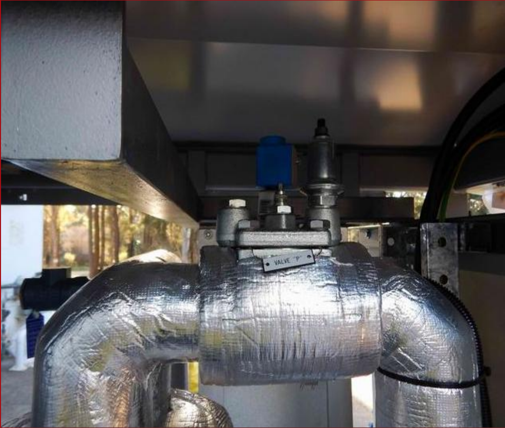
Danfoss regulating valve
