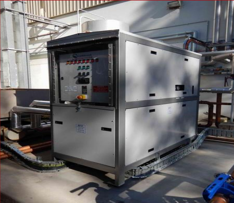
Integrated control panel
