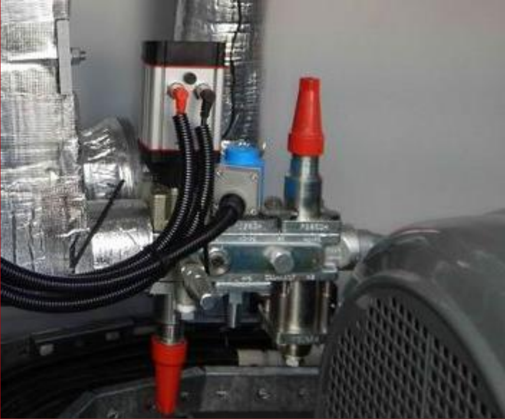
Ultra compact Danfoss ICF valve station
