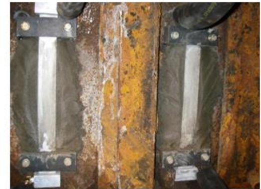
Freezing pipe attached at wall
