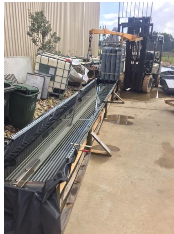
Figure 10 - Testing Condensing Tube Bundle @ 170bar with Dry Nitrogen.
