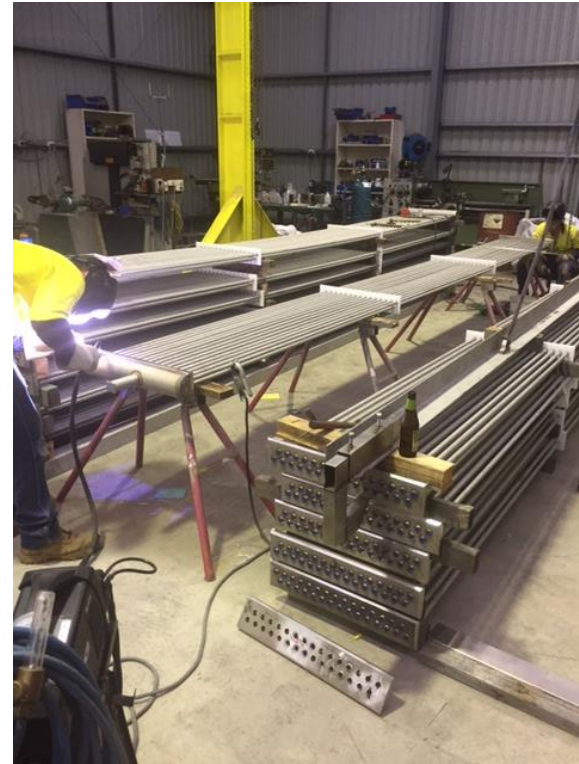
Figure 8 - Welding CO 2 Inlet Connection
