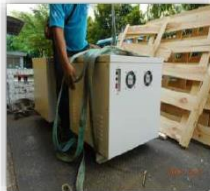
Unloading transformer for CO 2 CDU
