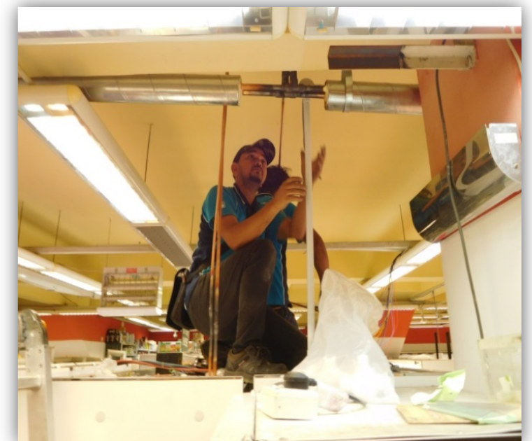
Piping work (inside store)
