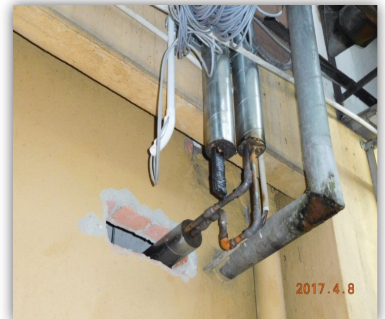
Piping work (Outside store)
