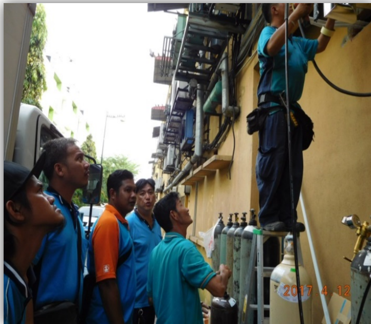
Piping work (Outside store)
