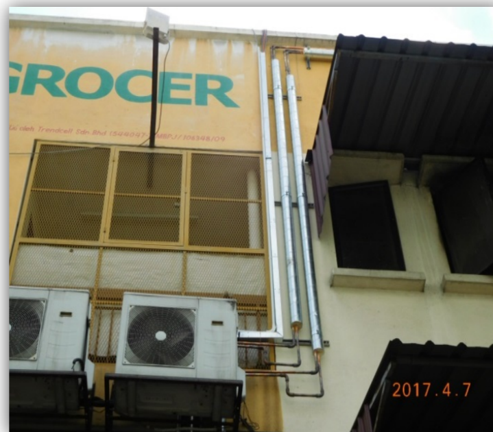
Piping work (Outside store)
