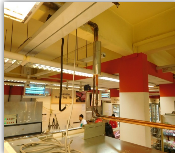
Piping work (inside store)
