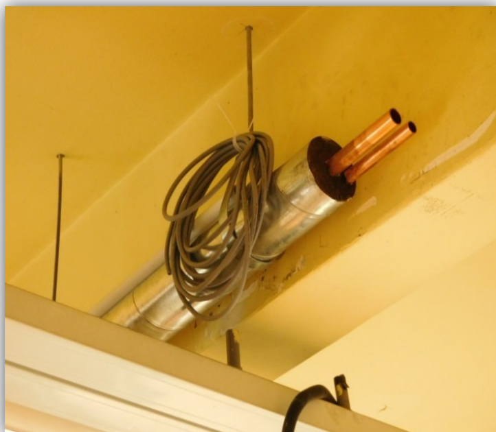
Piping work (inside store)
