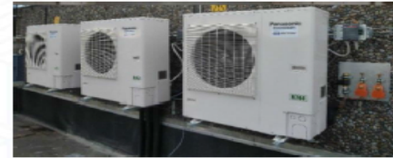
Condensing unit's on the roof.
