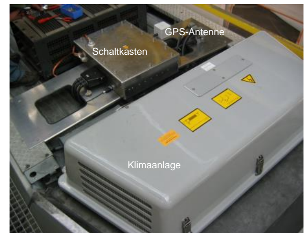
Roof installation on ÜSTRA tram 2005
