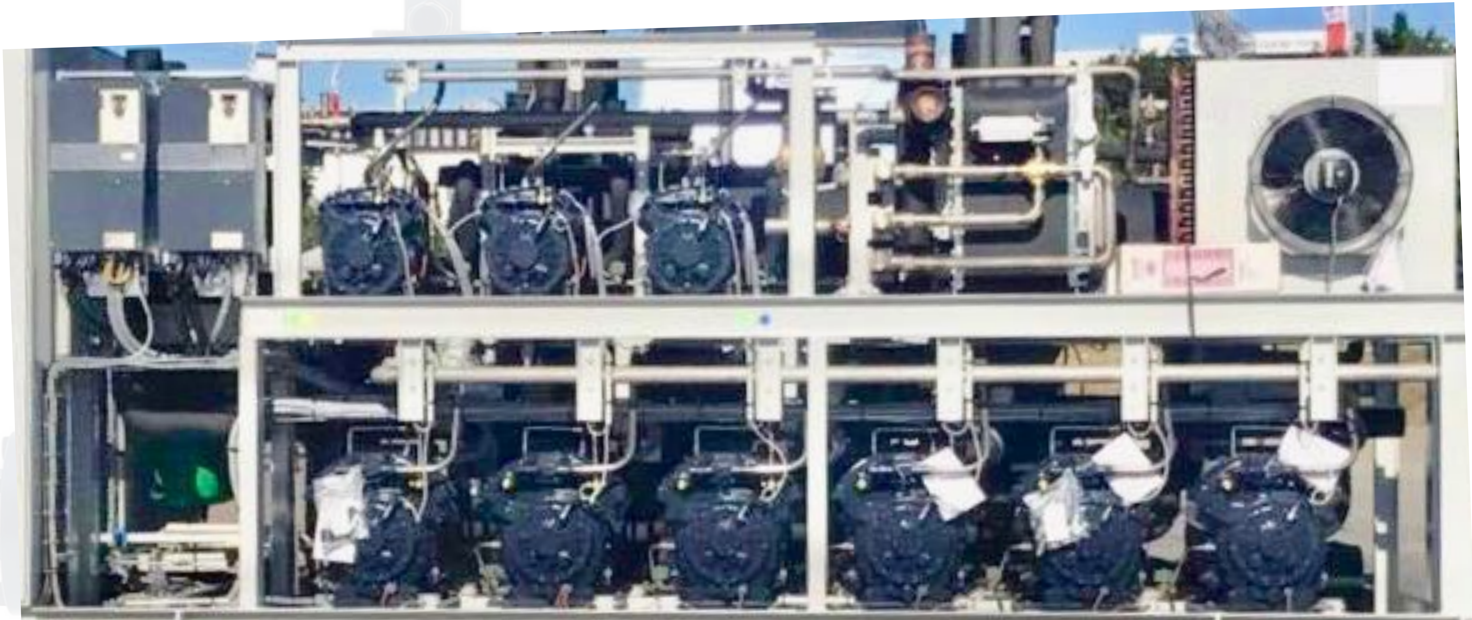
RACK WITH DORIN 6 CYL. TRANSCRITICAL COMPRESSORS 60 m 3 /h EACH courtesy PROFROID - GREEN & COOL
