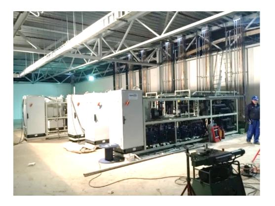
*C1: (L4+2)* 463kW @-5C HR 205kW (30/80C)
