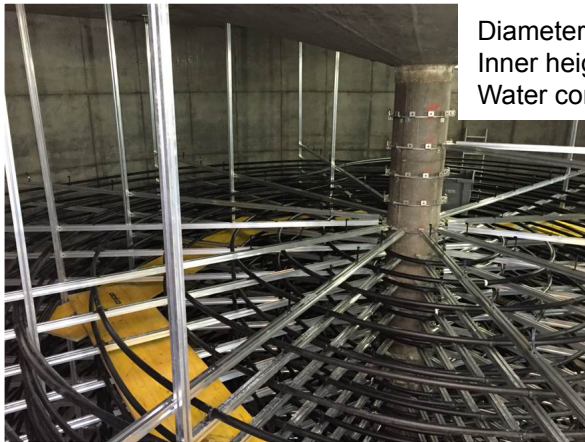
Laying of plastic heat exchanger tubes (32 mm x 2 mm) Cylindric cisterne of concrete
