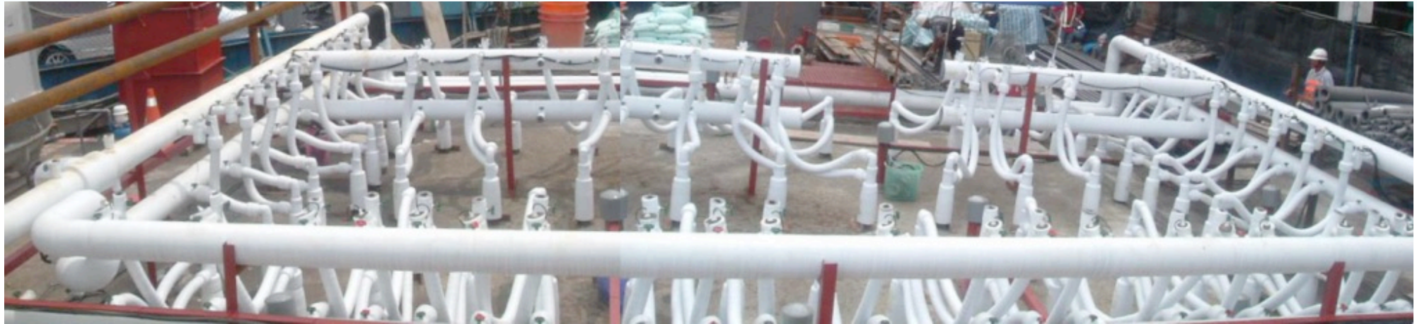
Freezing Pipe on Ground
