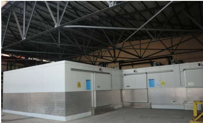
3 (-18°C) fish oil cold rooms in Shuangcheng factory
