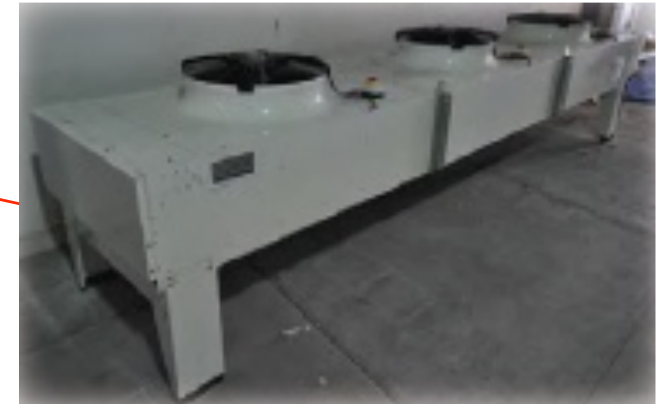
Gas Cooler/Condenser
