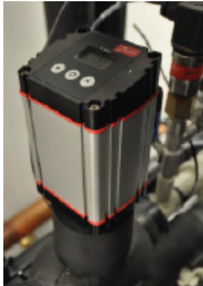
High Pressure Control Valve
