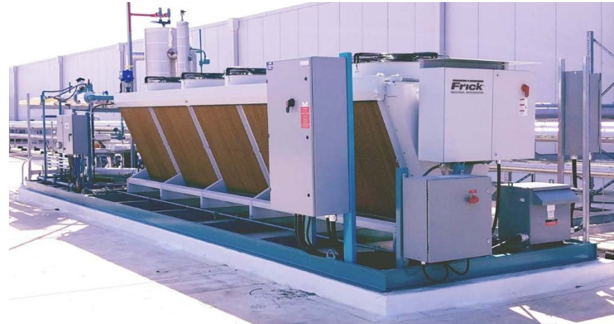
RDC #4 Setting on Roof Curb Servicing (4) Dock Evaporators
