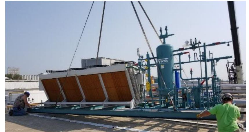
Adiabatic RDC Package for Expansion – Nebraska, Phase II
