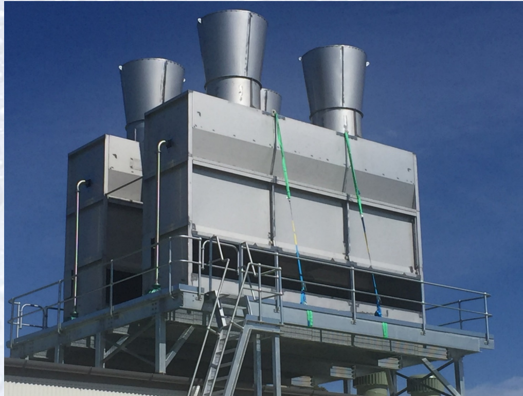
Figure 1: World's First Hybrid CO 2 Gas Cooler/Evaporative Condensers Installed at a Job Site in Sydney
