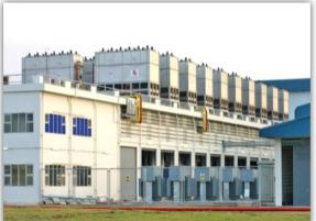
21 sets of SS Evaporative Condenser with total power of 18,000 HP, with total nominal heat reject of 50,000 kW
