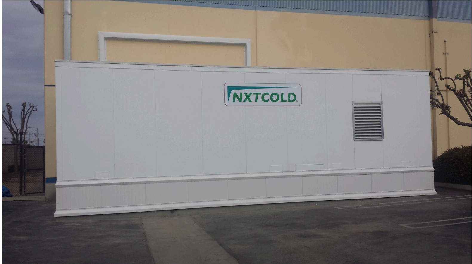
Complete Self Contained Ultra Low Ammonia Charge Refrigeration System 50 Tons Refrigeration : 25 Lbs. Ammonia
