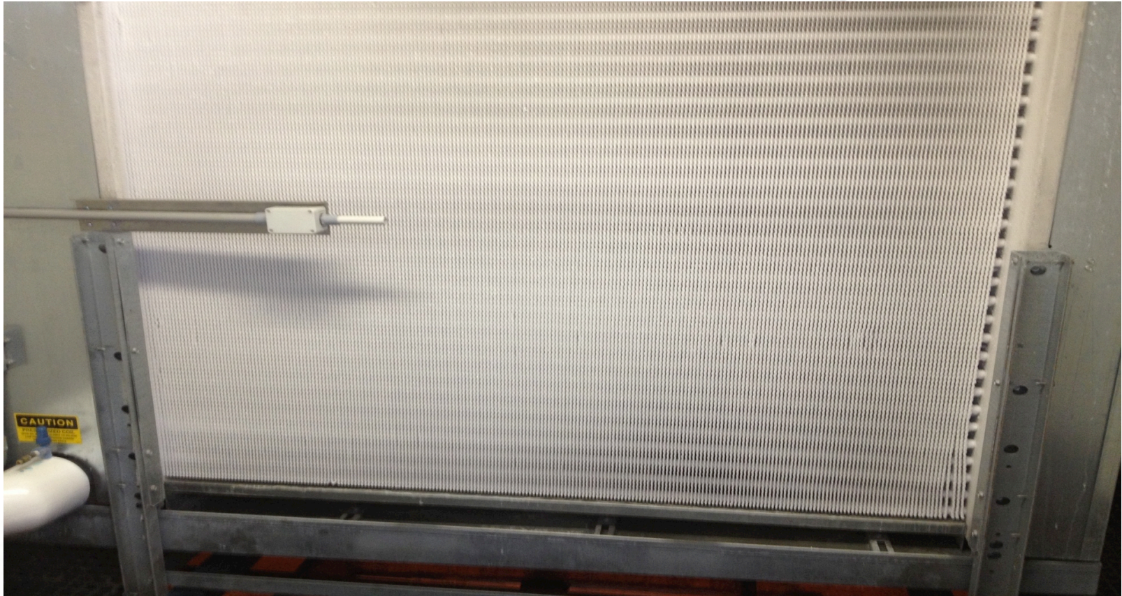
Evaporator Frost Pattern
