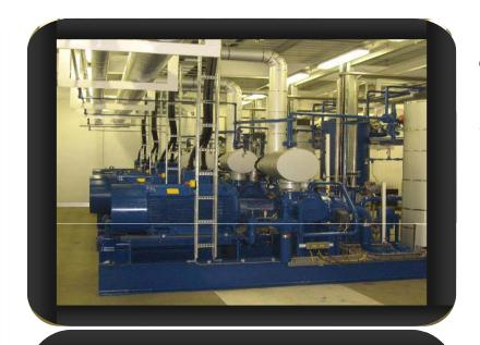
1.6 MW, 61°C, Process heating 2 x 1 stage 0.8 MW Systems
