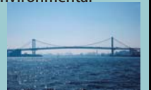
Materials provided by the Bureau of Port and Harbor, Tokyo Metropolitan Government
