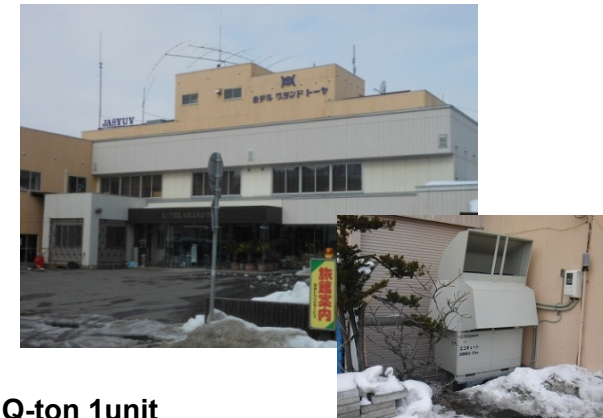
Q-ton 1unit Unvented cylinder 4000L
