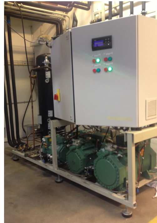
40+10 kW with CO 2 MT and LT dual temperature Max 5 compressors per unit
